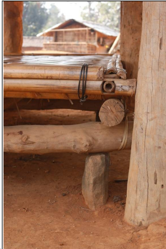
Figure 13: An elongated stone is used as a pillar to support the main frame of the house
