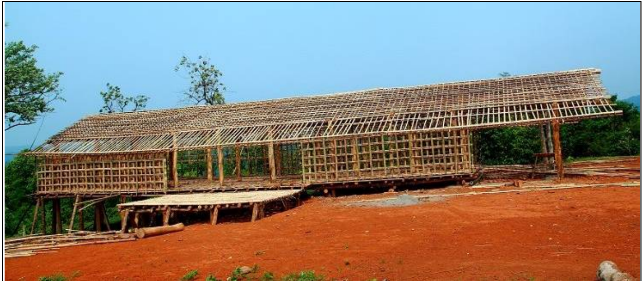
Figure 12: A nok achik being constructed (Photo credit: Semberthush Sangma)
