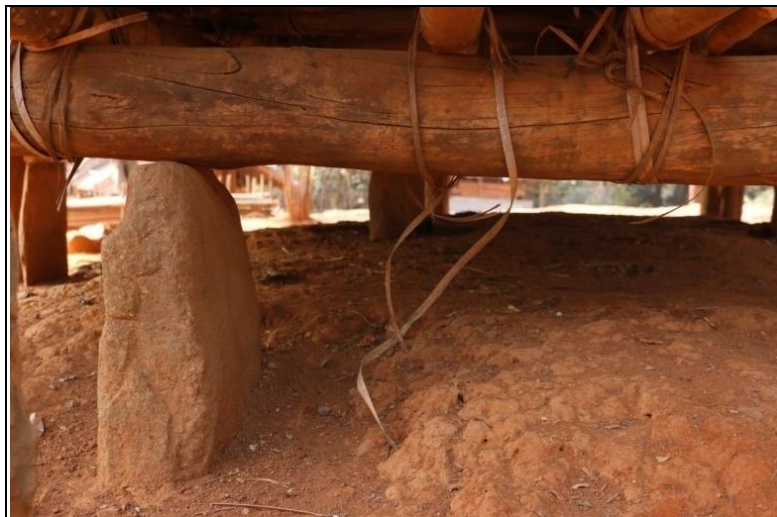
Figure 14: Another view of a stone used as pillar
