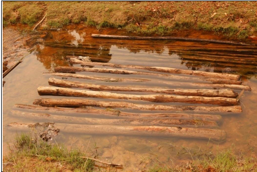
Figure 17: Wood being kept under water for days before construction
