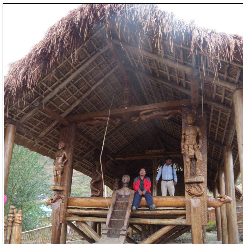
Figure 10: A view of the nokpante built at Naga Heritage Village, Kisama
