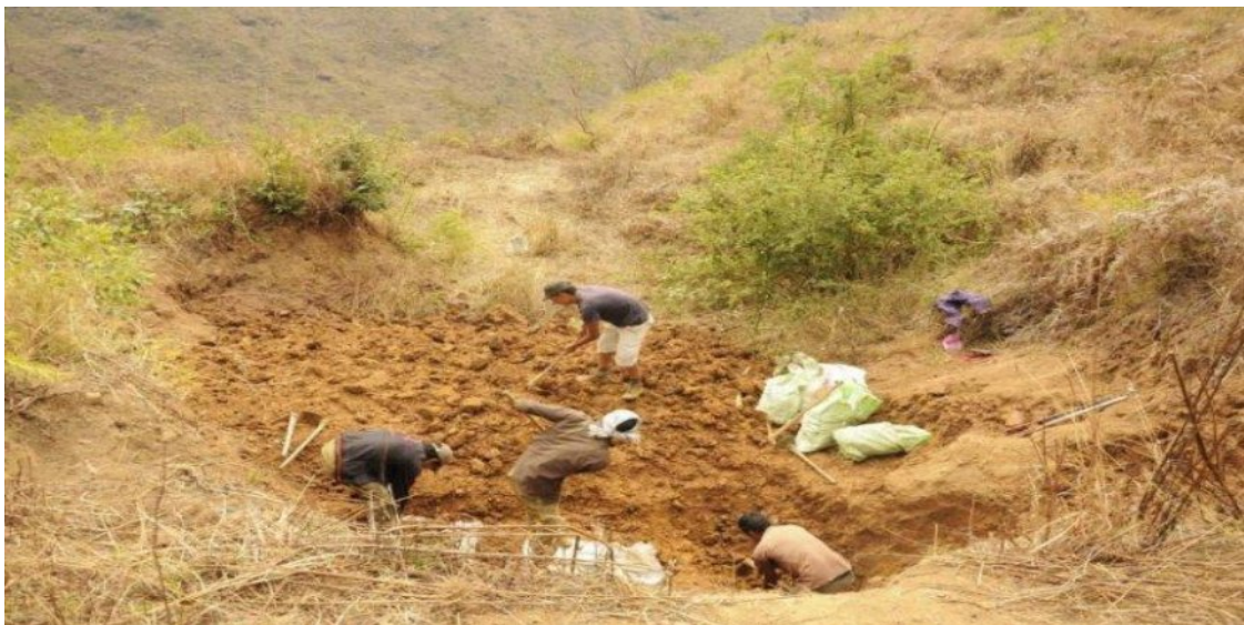
Figure 2: Kala Kaphung, where the lateritic soil is excavated for making Longpi Hampai.
