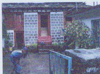
Local Stone Called Bhutti Dhunga Used For Construction
